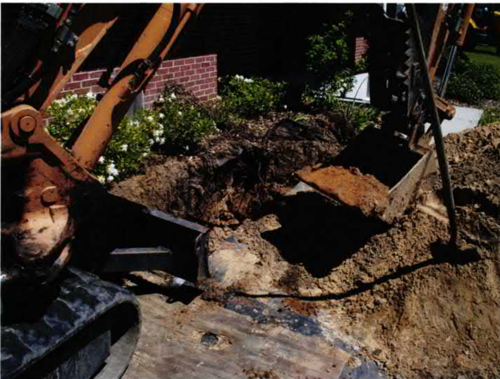
Picture 2: UST 849Dolphin excavation in progress.
